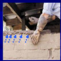
Preparing and using Mud as a mortar
